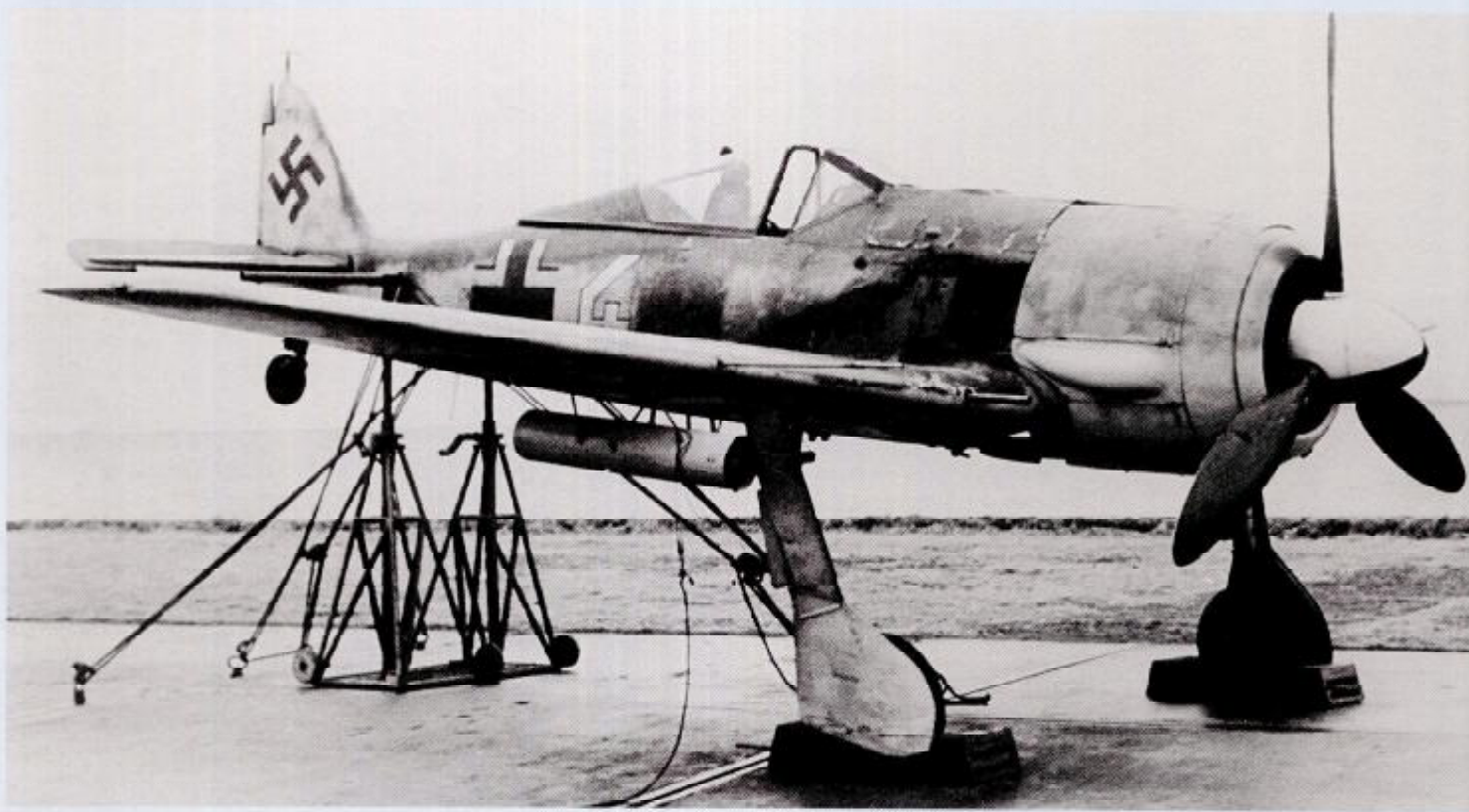
ABOVE: Fw 190A-5, W.Nr. 1372, 'White 4' of the weapons testing and evaluation unit, Erprobungskommando 25, was used to conduct firing trials with the 21 cm air-to-air mortar. Built by Focke-Wulf in Marienburg, it is believed the aircraft was with JG 1 before being transferred to Ekdo . 25. In this dramatic photograph, taken at Barth airfield, west of Stralsund on the north German coast in early 1944, a mortar is remotely fired from the aircraft for testing purposes and aimed across the waters of the Barther Bodden in the direction of Zingst.
