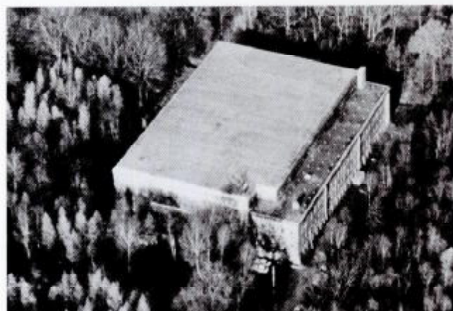
ABOVE: An aerial view of the immense, purpose-built divisional fighter control bunker at Arnhem-Deelen in Holland. Constructed largely of reinforced concrete to protect it from air bombardment, the building served as headquarters of the 1. Jagddivision under Generalleutnant von Döring from January to October 1943, when the Division was redesignated 3. Jagddivision under the same commander. The Division was responsible for the control of all day and night fighter units in north-west Germany, Holland, and parts of Belgium. Known as a 'battle opera house' because of its tiered seating system and artificial lighting, the building housed a team of experienced fighter controllers supported by auxiliaries and a sophisticated communications and reporting system.
