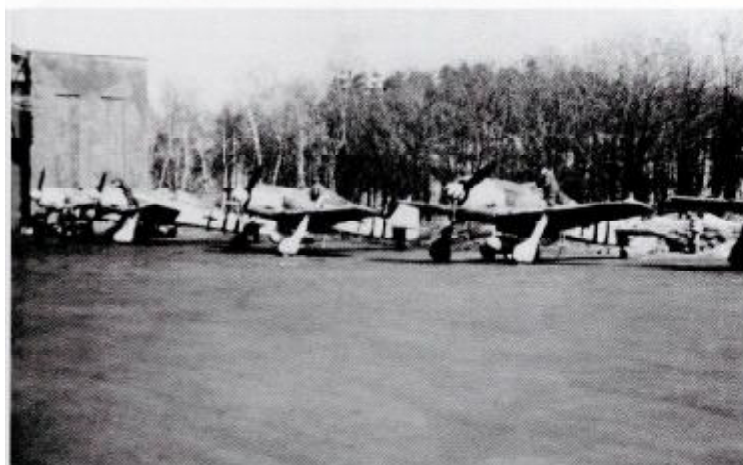
ABOVE: Ground personnel with the Fw 190s of Sturmstaffel 1 at Salzwedel in February or March 1944. All aircraft have been fitted with 300 litre drop tanks and the spinners have been painted with a black and white spiral.
