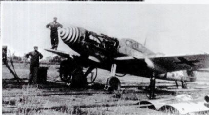
THIS PAGE: Groundcrew of III./JG 1 work on some of the the Gruppe's Bf 109 G-6/R-6 aircraft. All machines have spiral spinners and are armed with MG 151 cannon in underwing gondolas.
