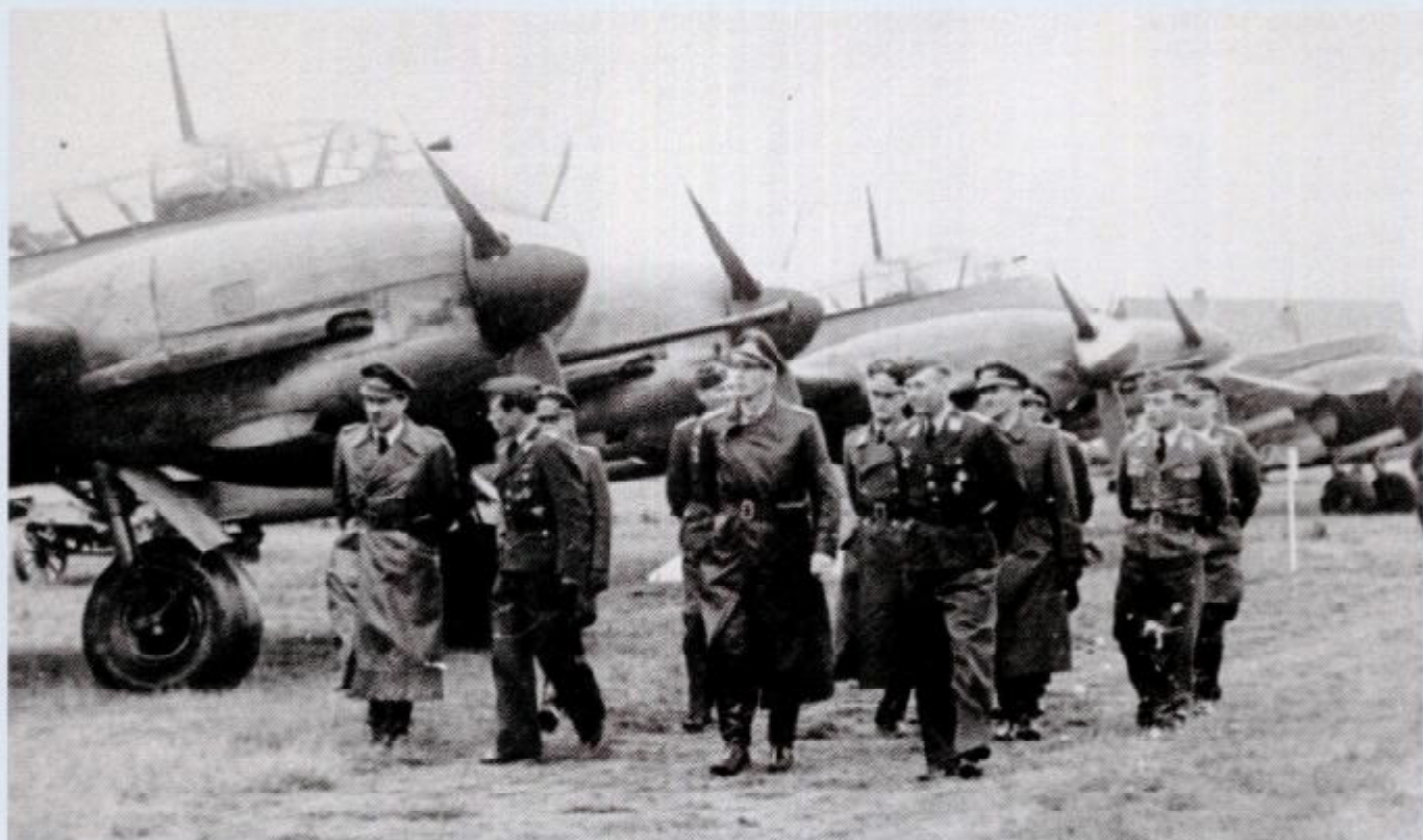
BELOW: Galland (far left) makes his way past the two Me 410 Zerstörer of Erprobungskommando 25. Note the aircraft are fitted with 3.7 cm Flak 18 cannon which the unit was evaluating as a weapon to combat daylight bomber formations. Also seen are, from the left, Geyer speaking to Galland, Hptm. von Kornatzki (Sturmstaffel 1), Oberst Hannes Trautloft (soon to be appointed Inspector of Day Fighters), Oberst Günther Lützow (commander of 1. Jagddivision), Oblt. Reebman (Ekdo. 25), Oblt. Edu Neumann (Stab. G.d.J.), Stabs. Ing. Öhlkers (Ekdo. 25), and Oblt. Frodl (Ekdo. 25).
